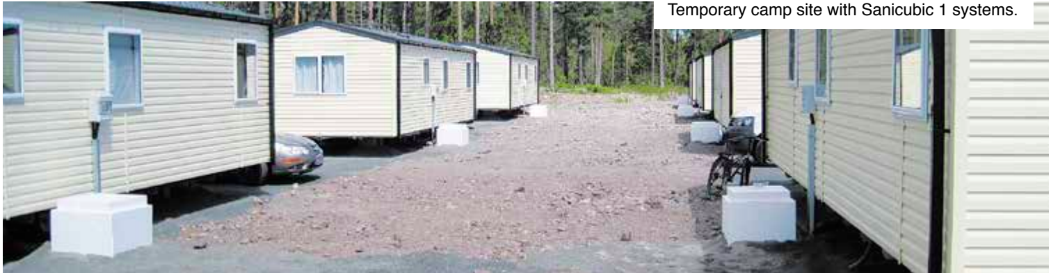
Temporary camp site with Sanicubic 1 systems.
