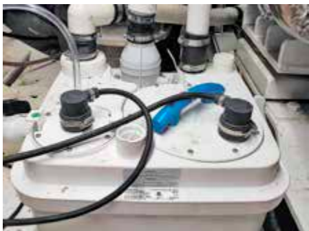
Inside the RV MANTA's mechanical room, showing the Sanicubic 1 and the 1.5-inch PVC piping to two of the Sanicubic 1's four input ports.
