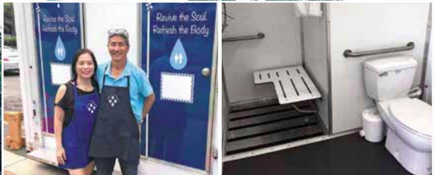
Inside the Revive + Refresh trailer's handicap-accessible bathroom, showing the Saniflo Sanibest Pro grinder system.
