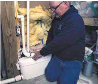
Plumbing contractor adjusts his Saniaccess3 macerator from Saniflo.
