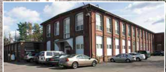
Renovated Remington Rand building in the city of Middletown, CT
