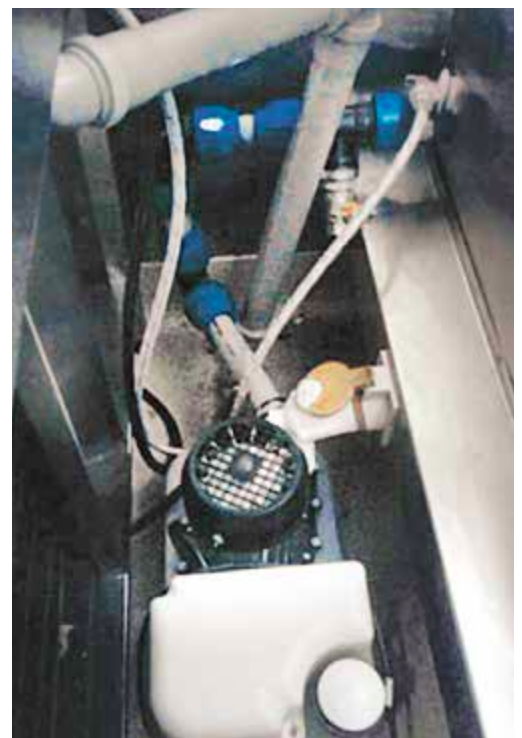
Pump installation behind oven
