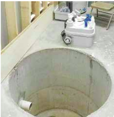
The Sanicubic 2 grinding system from Saniflo pre-installation in the underground pit.
