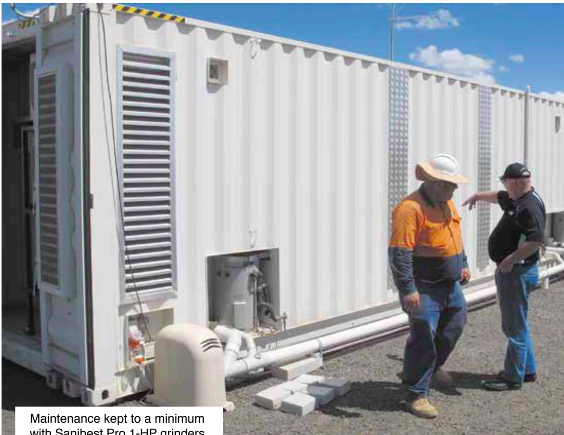
Fixtures from a complete bathroom are drained into the Sanibest Pro
