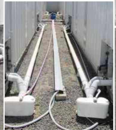
Sanibest Pro units pump the shredded waste over 100 feet horizontal
