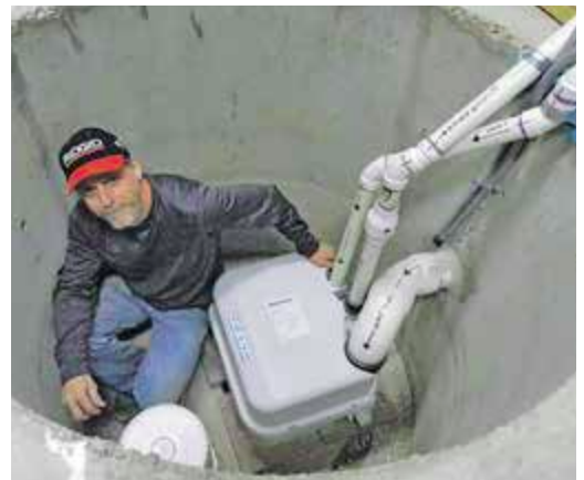
The Sanicubic 2 grinding system from Saniflo pre-installation in the underground pit.
