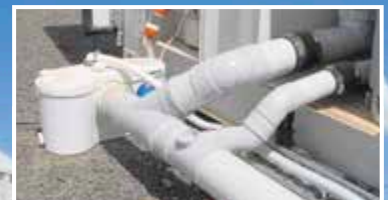
Fixtures from a complete bathroom are drained into the Sanibest Pro
