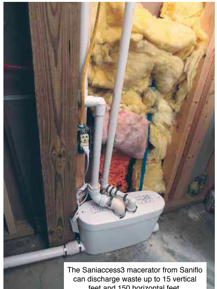
Plumbing contractor recently made the decision to install an above-floor plumbing system from Saniflo in his log cabin's basement.
