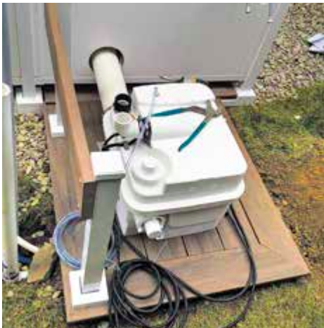
The one-horsepower Sanicubic 1 grinding system handles wastewater from a toilet, sink or shower in the outdoor enclosure
